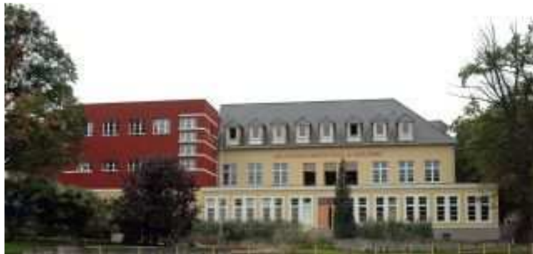
View from the main street and tram stop
